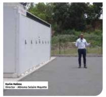
Located near Longoni Bay, this installation is made up of batteries that store energy in off-peak hours and re-inject it later during peak consumption. Albioma makes the plant available to the network operator, Énergie de Mayotte (EDM), which determines its production programme. It works like an energy tank, which EDM can fill and empty to optimise its production resources and ensure the balance between consumption and production. Albioma is the owner and operator of this plant.
