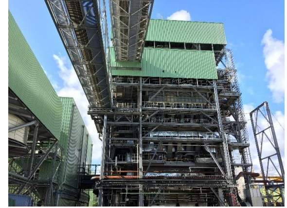
Boiler and biomass conveyor
